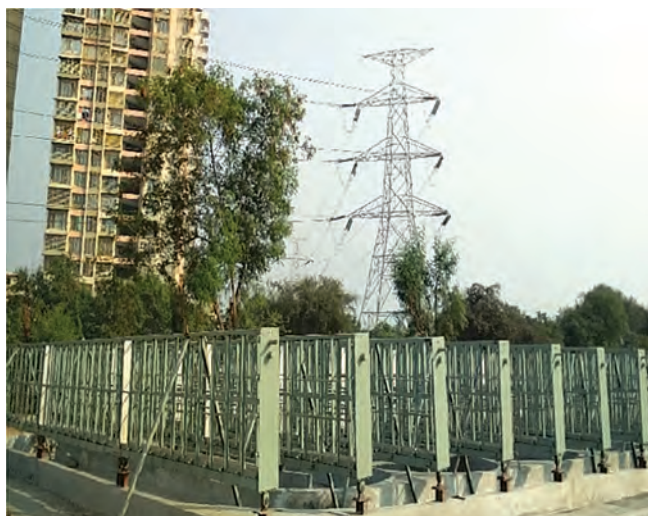
Installation of 100,000 L algal growth system at Mumbai coastal site
